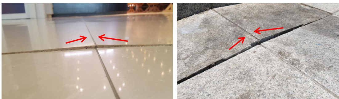
< Expansion problem case: Left: Engineered stone, Right: Natural stone >
